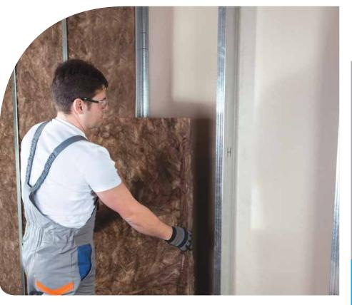
MineralPlus IPB 037 Partition Wall Insulation Slab
